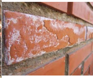
EFFLORESCENCE & SPALLING
